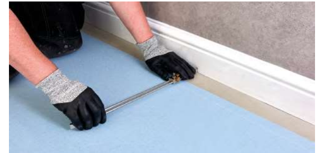
Figure 3.2 Scribing the wall profile
