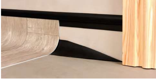
Figure 3.7 Taper towards a doorway
