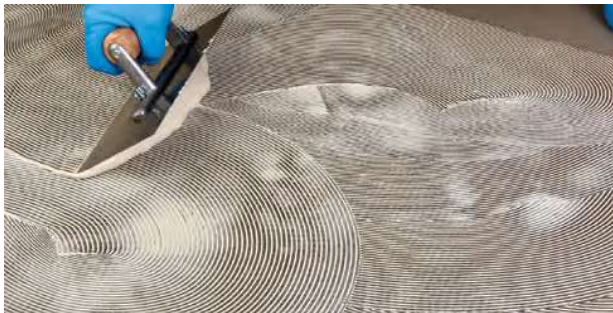
Figure 3.6 Spread the adhesive
