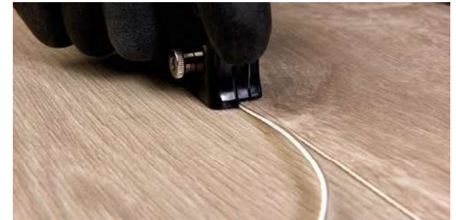
Figure 3.5 Cutting in the seams
