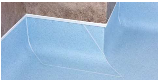
Figure 3.9 External corners 'wrap around method'
