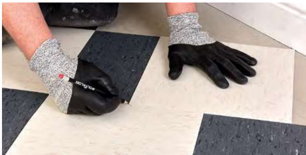
Figure 4.7 Marking the perimeter tiles (diagonal cut)
