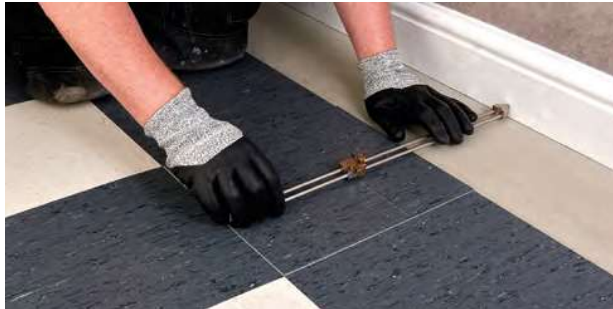
Figure 4.6 Measuring a tile using a scriber
