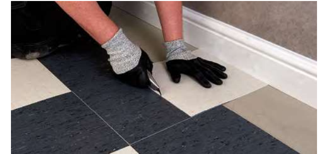
Figure 4.5 Measuring using an overlapping tile
