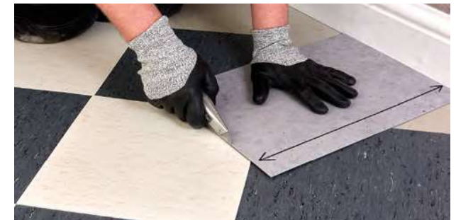
Figure 4.8 Cutting the perimeter tiles (diagonal cut)
